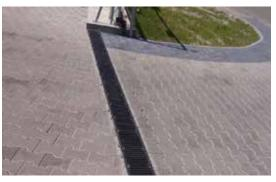
Trench drain 150F with cast iron grating
