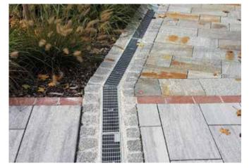
Trench drain 100/V line with pressure-locked grating 30/10
